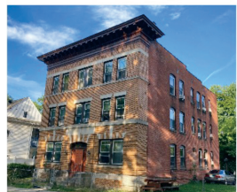
33 Bethel Street • Built 1920 2, 2-Bed units, 4, 3-Bed units
