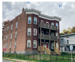
243 Capen Street • Built 1915 6, 3-Bed units
