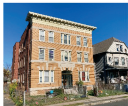
34 Pliny Street • Built 1920 4, 2-Bed units, 2, 3-Bed units
